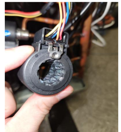
Remove & Inspect EEV Coil for Rust or Foreign Object
